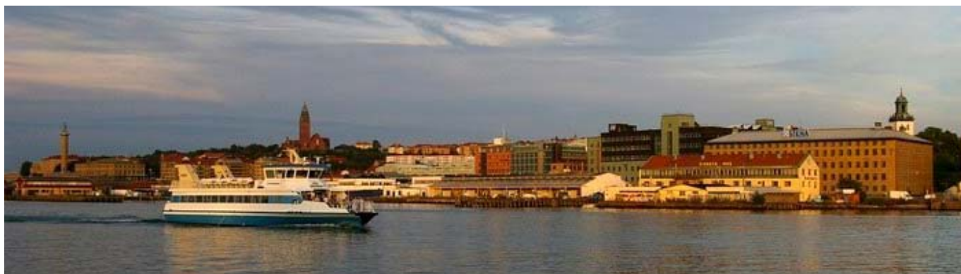
The world's northernmost district air conditioning
